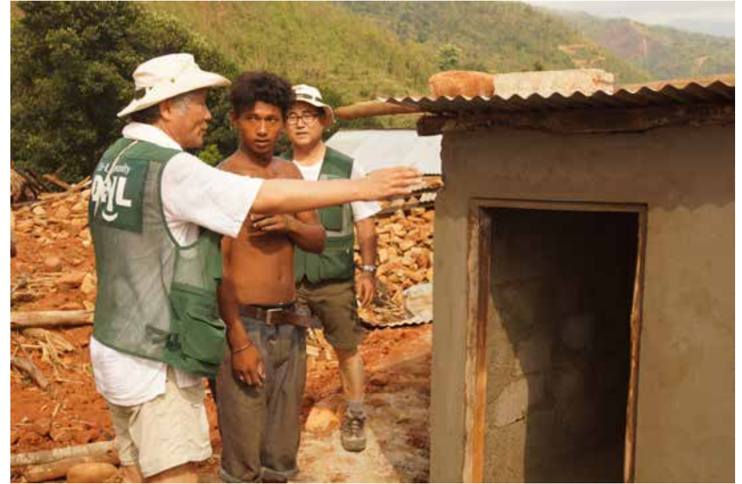
Public Village Restroom Construction Site
