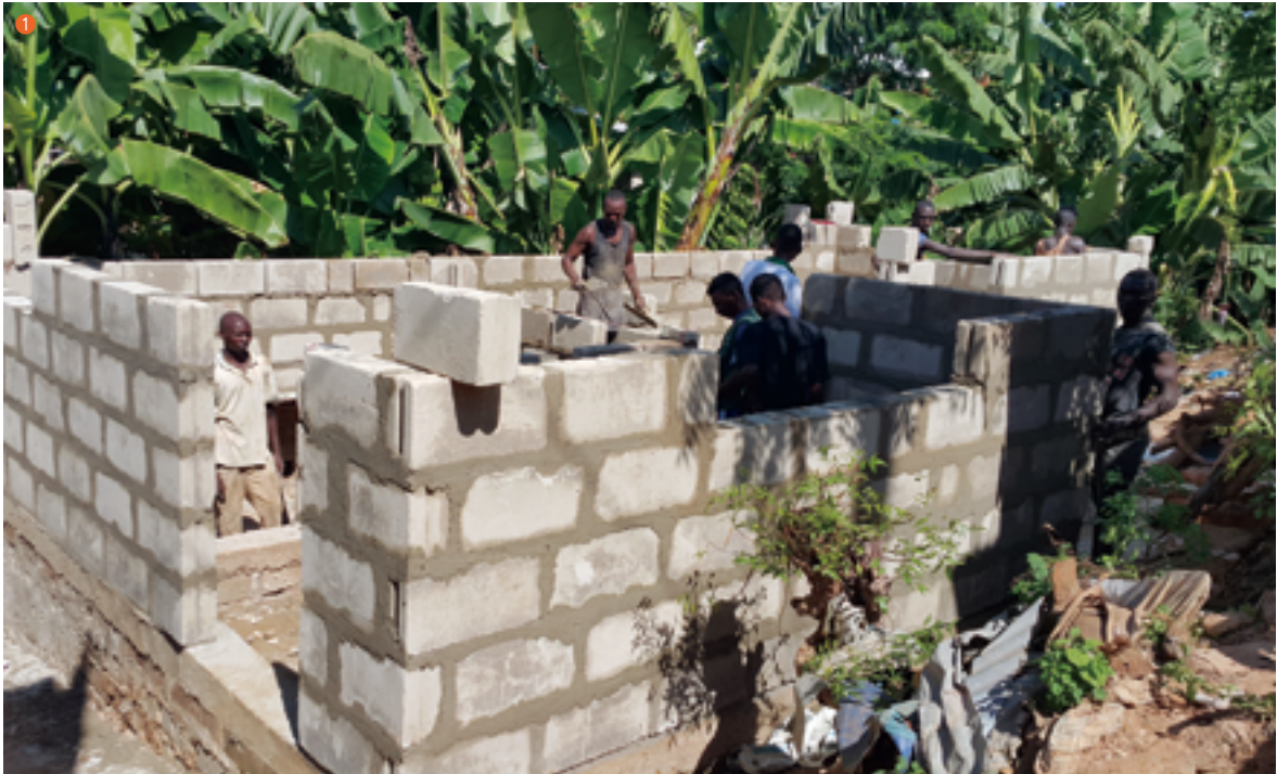
1 Construction on Sophia's new home
